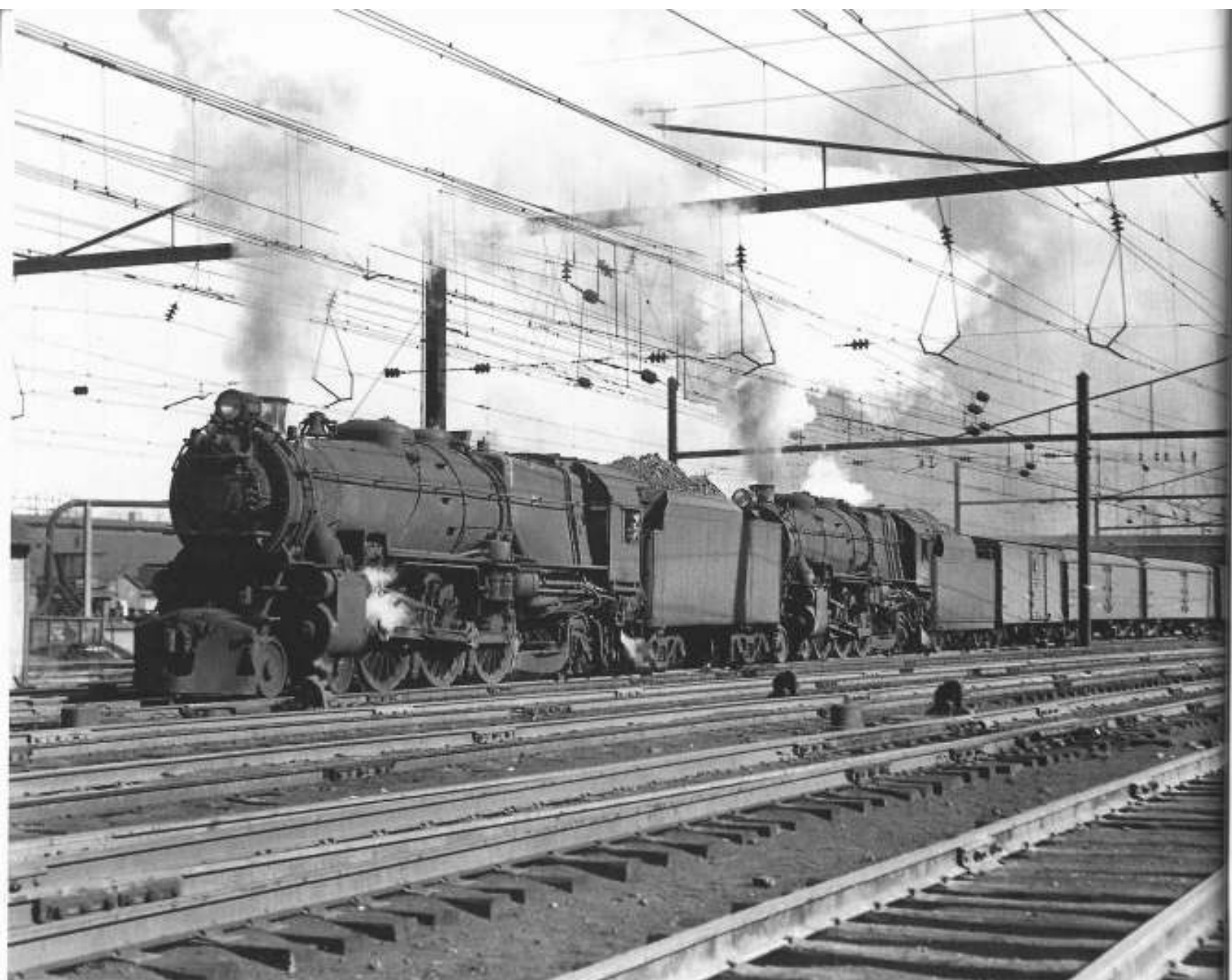
Two K4s Pacifics accelerate a mail and express train, brought in from the east by a GG1 electric, out of Harrisburg in March 1946. The T1 was intended to end doubleheading on PRR's "Blue Ribbon Fleet" of east-west passenger trains, and to be the equal of a GG1.
